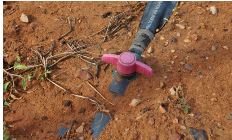
Vanne semi ensevelie
